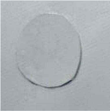
Place the patch on the damaged area and press down firmly. Let the glue sit for 2-4 minutes until it appears tacky. If glue does not hold, heat patch with a hair dryer.
